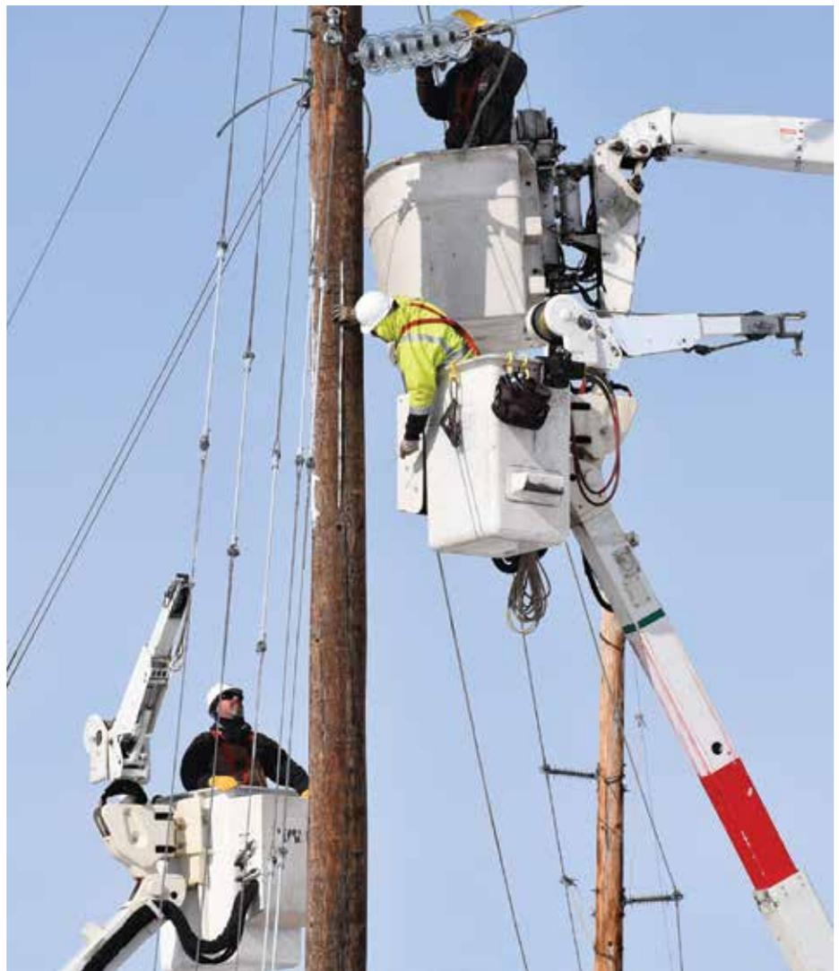
limiting potential injuries from burns and sparks. Insulated and rubber gloves are worn in tandem to protect them from electrical shock. While the gear performs a critical function, it also adds additional weight and bulk, making the job more complex.
